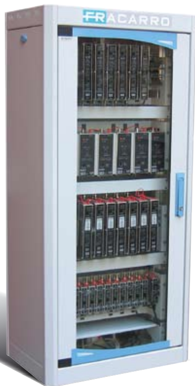
19 inch rack installation
